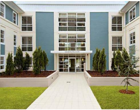
For the higher units, the Vantage Series 613 MAGNUM™ Double-Hung windows were used for their durability and ability to complement high rise applications. This particular double-hung window is robust and hardwearing, making it the perfect fit for apartments. The sashes fully bypass each other to allow cleaning of the glass from the inside which is the perfect solution in high rise applications like the residences on Breakfast Point.
